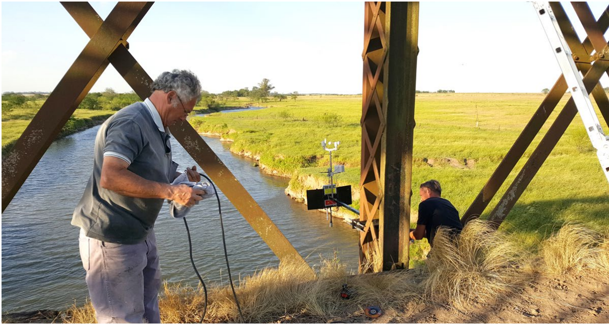
Installation of the nodes at Conesa bridge, Buenos Aires
